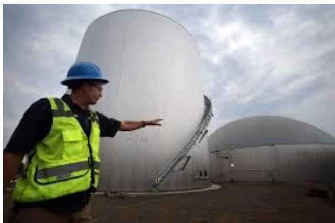
Figure 2-2: Photo of JC-Biomethane's Anaerobic Digestion Facility in Junction City, Oregon
