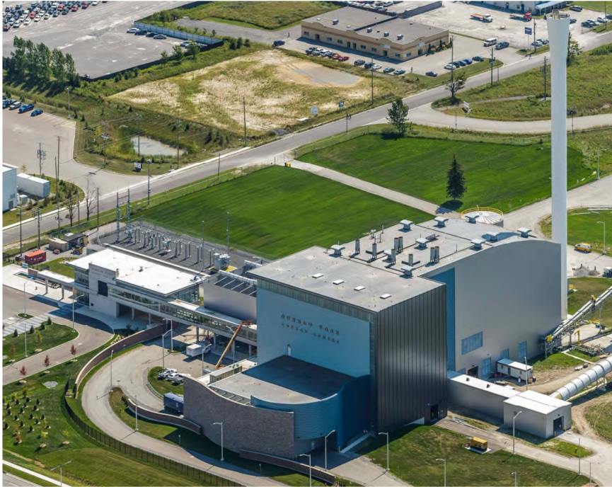
Durham Region Waste-to-Energy Facility; Ontario, Canada
