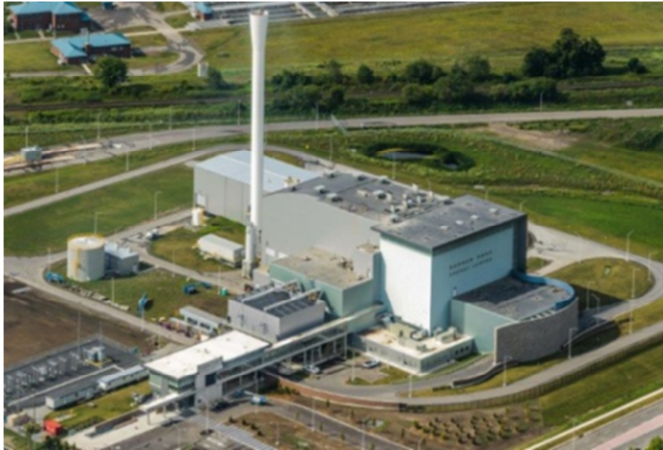
Figure 2-4: Photo of the 480 TPD Durham-York WTE Facility in Ontario, Canada
