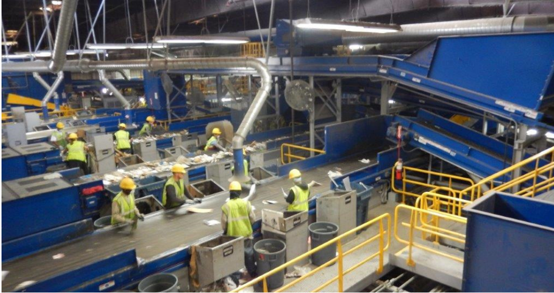
Newby Island Resource Recovery Park; San Jose, CA
